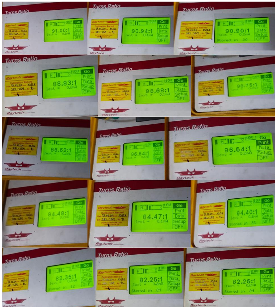
Figure 6. Raytech Transformer Turn Ratio Measurement Coil 1 (Left side - 5 times); Raytech Transformer Turn Ratio Measurement Coil 2 (Center side - 5 times); Raytech Transformer Turn Ratio Measurement Coil 3 (Right side five times)
