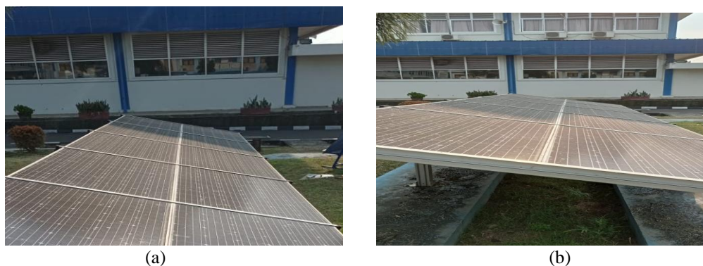
Figure 3. Shading Solar Panel Conditions (a) In the morning and (b) In the afternoon (right)
